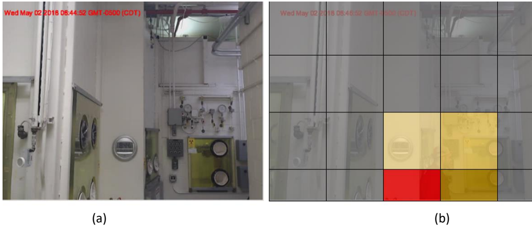
Figure 3. (a) Camera image from unit #1114 before motion (event) detection on May 2, 2018, 08:44:52 GMT and (b) pixel-frame-based motion (event) detection on May 2, 2018, 08:46:52 GMT. (Colors indicate differences in changes of image intensities in successive images.)
