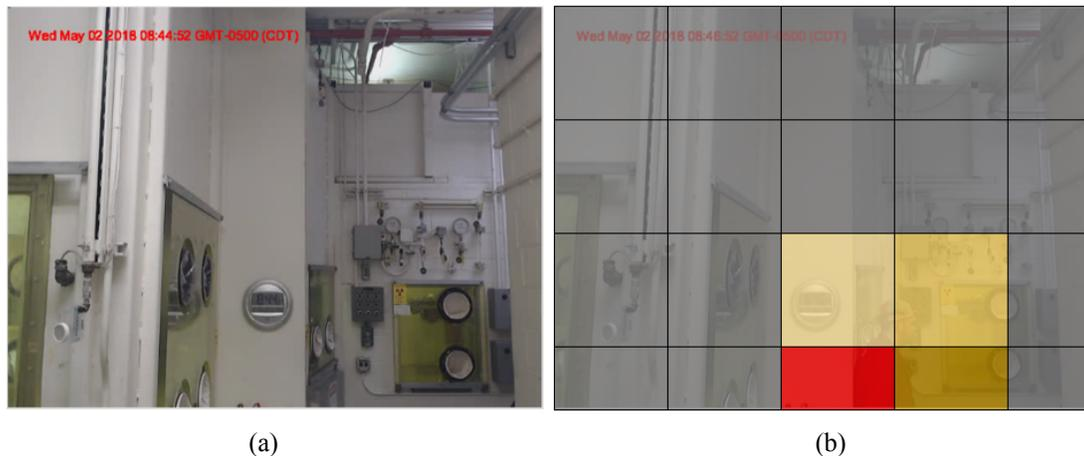
Figure 5. (a) Camera image from unit 1114 before motion (event) detection on May 2, 2018, 08:44:52 GMT and (b) pixel-frame-based motion (event) detection on May 2, 2018, 08:46:52 GMT. (Colors indicate differences in changes of image intensities in successive images.)
