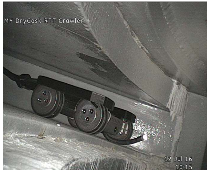
FIG. 22. Canister exterior surface inspection (courtesy of 3Y).
