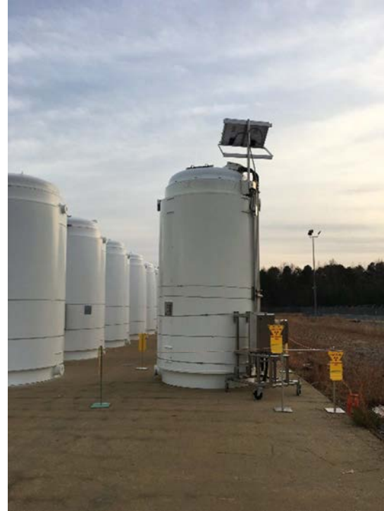
FIG. 5 Metal cask scheme for dry storage of spent fuel assemblies (left); TN-32B example (right) (courtesy of Orano NPS).
