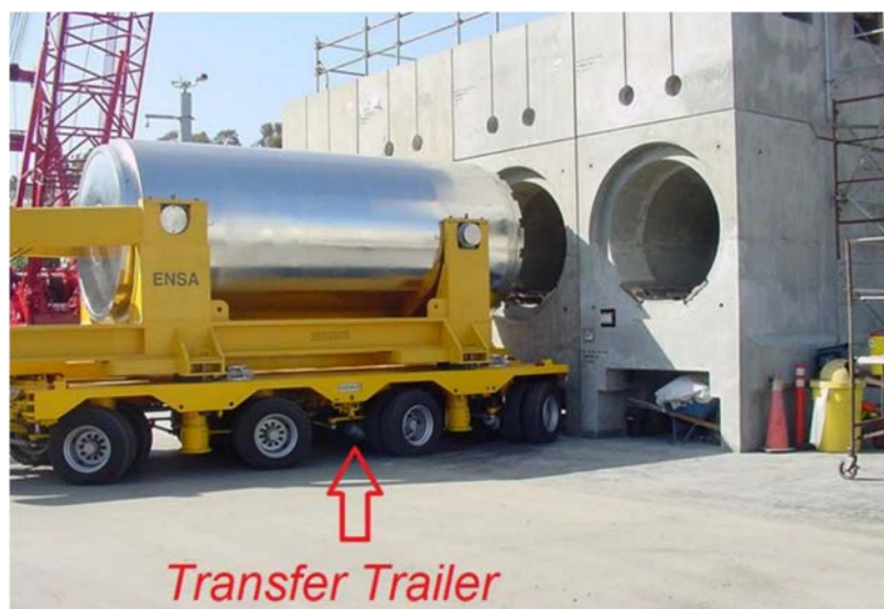
FIG. 9. Loading of a horizontal storage module (courtesy of South California Edison).
