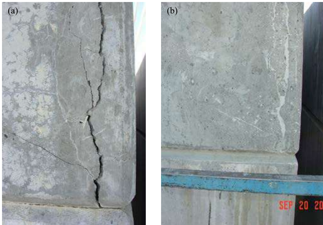
FIG. 42. Concrete horizontal storage module crack repair (courtesy of U.S. NRC).
